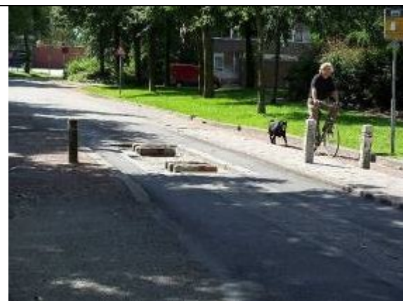
Groningen suburban bus/cycle gate
