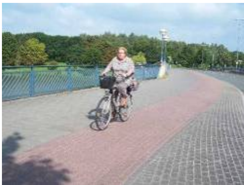
Cycle path flush with pavement
