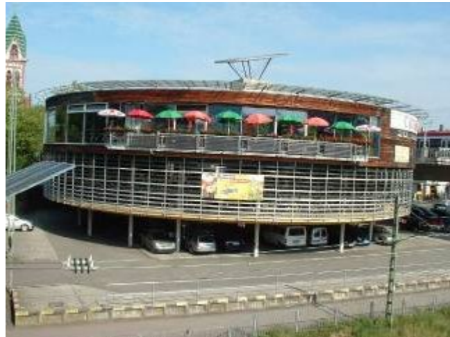
Cycle park at main railway station
